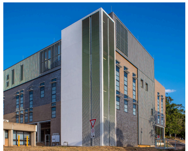
Figure 2.18 - NW Corner (stage 2)
