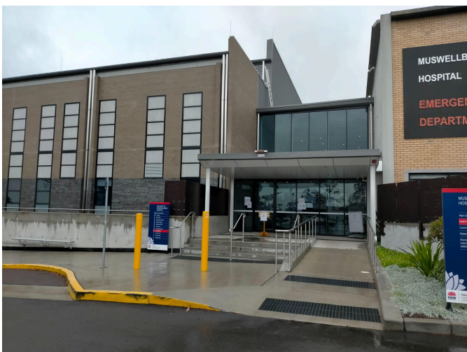
Figure 2.17 - Main Hospital Entry (stage 2)
