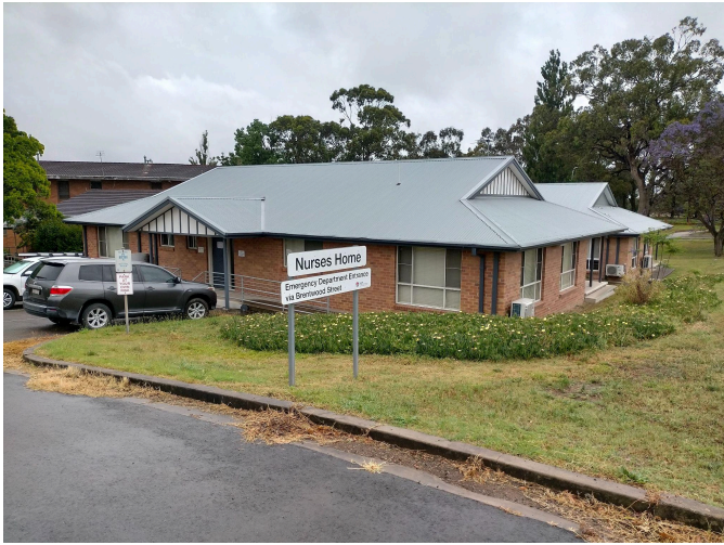
Figure 2.13 - Existing staff accommodation buildings
