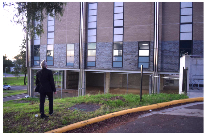
Figure 2.12 - Stage 2 lower ground undercroft
