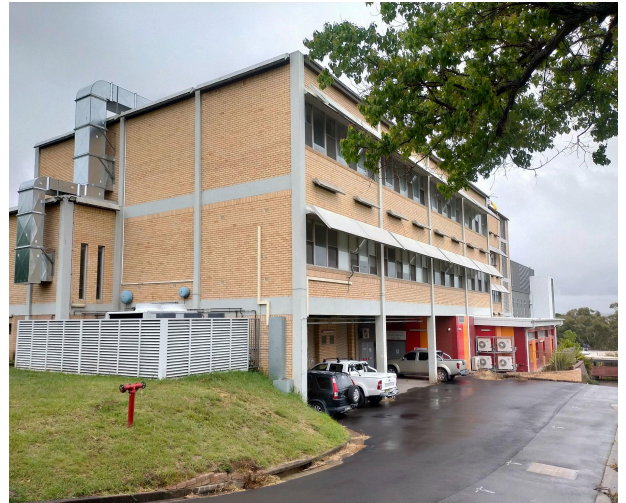
Figure 2.14 - Main hospital building (NE cnr)
